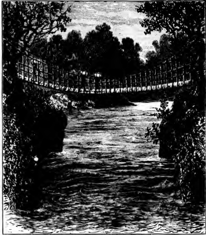
SUSPENSION BRIDGE ACROSS THE E. ITURI.
